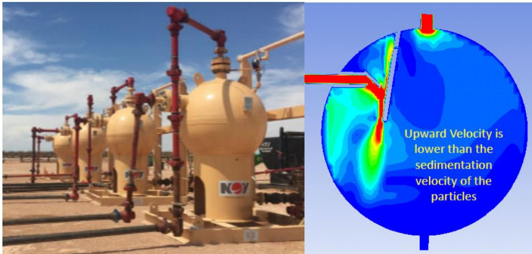
The main features from the Sand Hog, including the inlet pipe stinger and the angled baffle plate, are both present. Although Sandtinel has not modeled NOV spheres in detail, it is expected that the behavior would be very similar to a Sand Hog on the basis of these features. There are no components to develop an effective Vapor Lock, nor to create a secondary pass at sand removal through retention time. Storage in the bottom hemisphere will also be limited.
